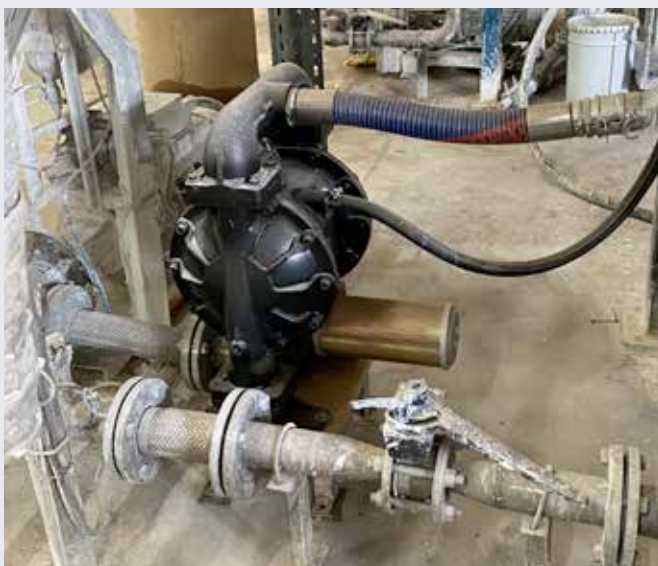
High suction lift reduces pump delivery.
