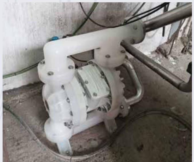
High fluid viscosity reduces pump delivery.
